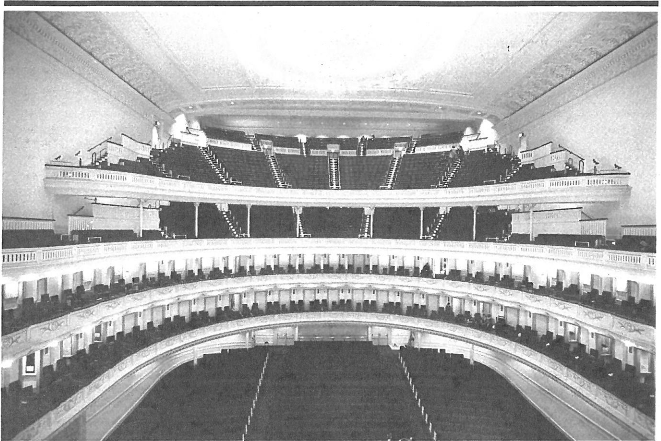
Air-delivery troffers and the large ducts they require are concealed in the ceiling of the main hall. The 2816 seats are divided into the following sections: parquet (bottom), first-tier boxes, second-tier boxes, dress circle, lower balcony, and upper balcony.
