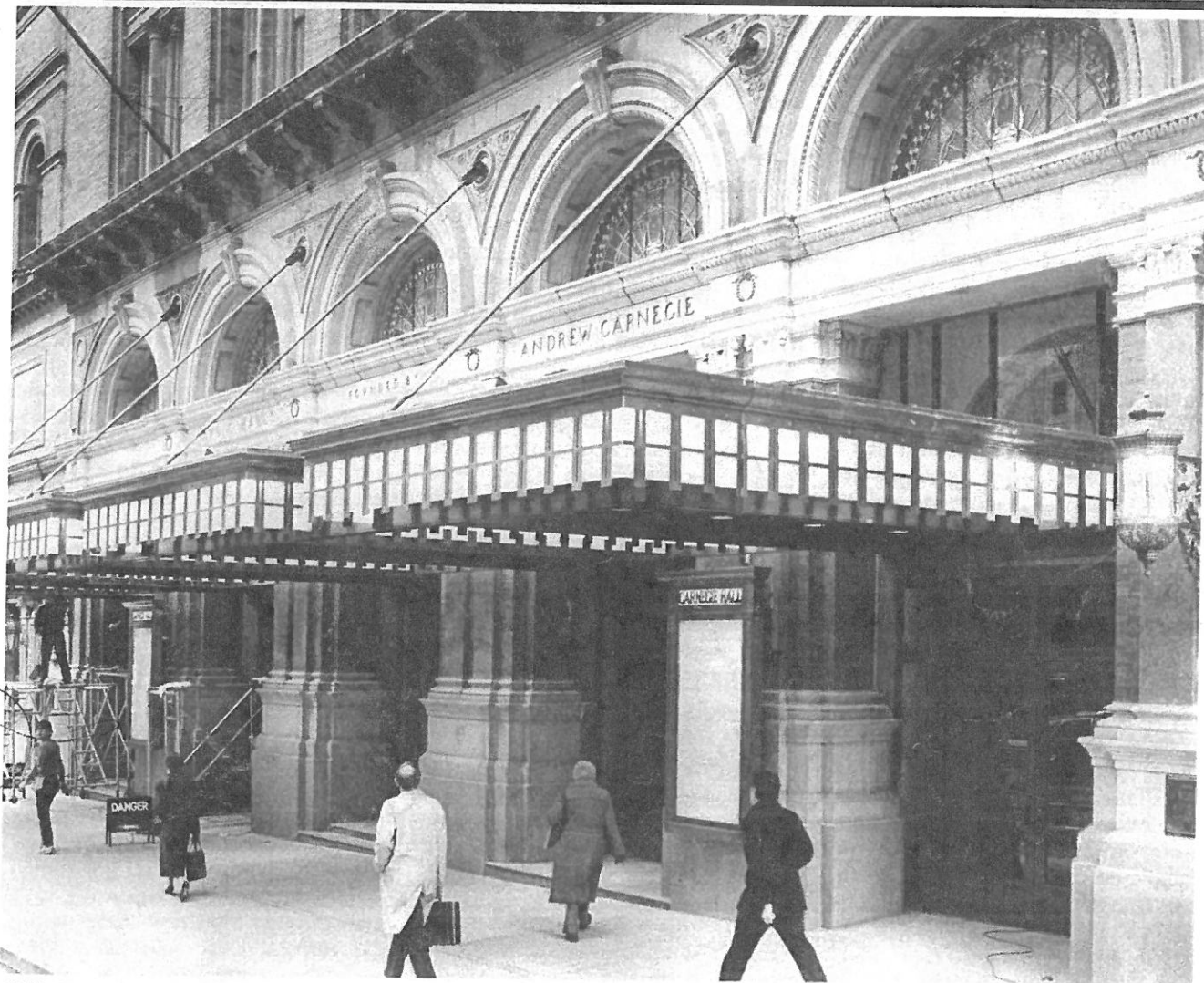
With its new air-conditioning system installed, Carnegie Hall will be able to operate year-round for the first time.
